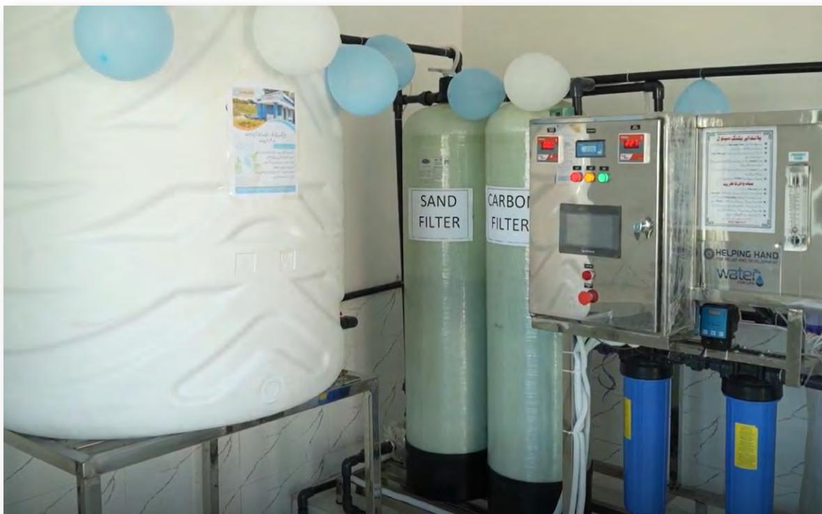
Reverse Osmosis (RO) is a water purification technology that uses a semi-permeable membrane to remove ions, molecules, and larger particles from drinking water. In the RO process, water is forced through the membrane under pressure, leaving behind contaminants such as salts, heavy metals, and other impurities. This method is highly effective in producing clean, safe drinking water, especially in regions where groundwater contains high levels of salinity or pollutants.
