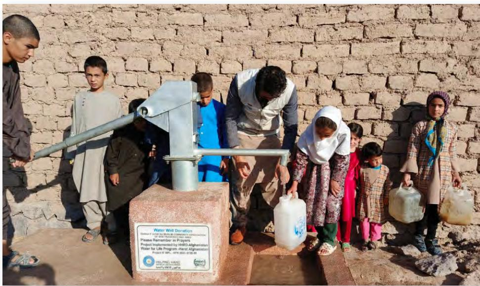
Afridev pumps are ideal for rural communities relying on underground water sources, providing an affordable and efficient solution to meet the water needs of low-income families. These durable, easy-to-install, and maintain suction hand pumps, made from cast iron, require no specialized components or expertise. HHRD delivers Afridev hand pumps in Afghanistan and Pakistan.
